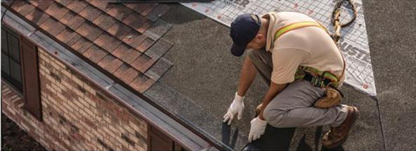
A shingle starter strip is an important part of a residential roofing system. It plays a critical role in reducing the risk of shingle blow-off along the eaves and rakes of the roof. It provides a base under the shingle at the eaves, helping the roof shed water efficiently. As its name implies, every asphalt shingle roof will start with this shingle.
